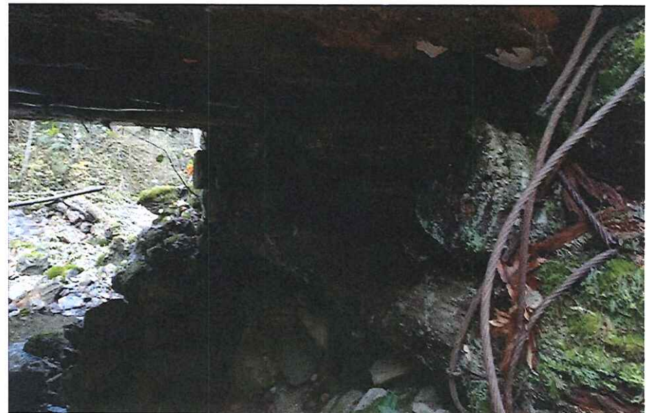
CK2254 Right Abutment
